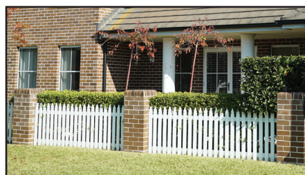
Figure 2.14.3. Face brick piers with picket
