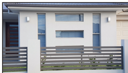
Figure 2.14.2 Front fencing with infill panels
