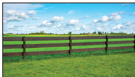
Figure 2.14.5. Dressed Hardwood posts and rail fence.
